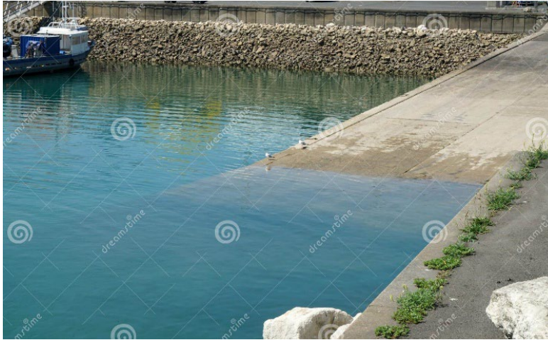
Figure 5-4 Example of slipway arrangement for vessel launch and recovery. Source: Dreamstime
