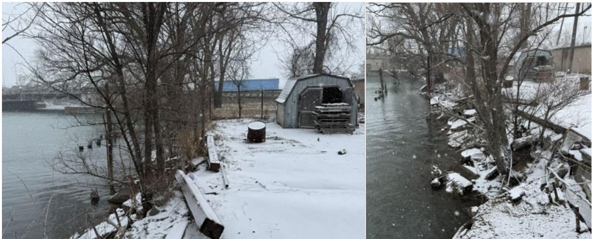
Figure 10-8 Photos of revetment at Western end of the site (Ramboll site visit Jan 2026)
